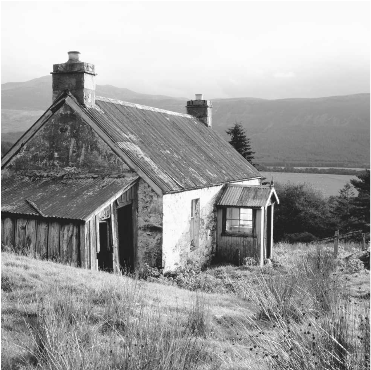
A small house in Gorstan. The poor quality of housing is a concern in both urban and rural areas.
